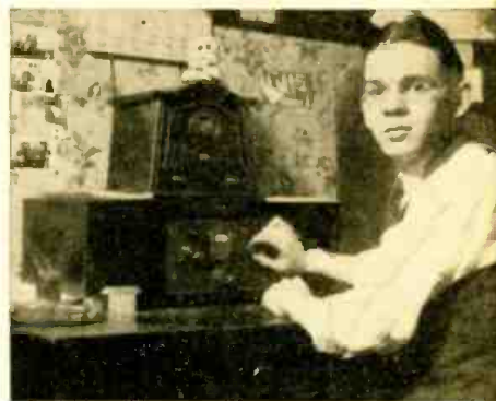
Mr. Whitmer's efficient looking station.
